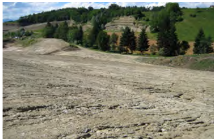
Remblai, phase I
